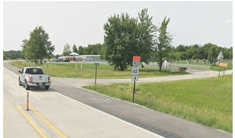
BEATTY ROAD EXISTING CONDITIONS
