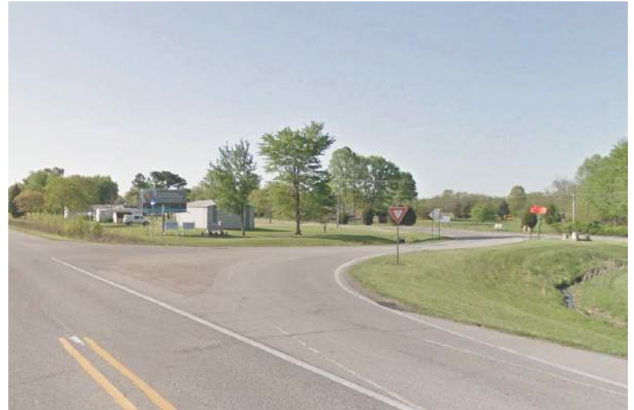
SHORT STREET EXISTING CONDITIONS
