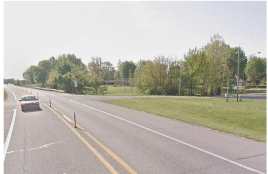
FRONT STREET EXISTING CONDITIONS
